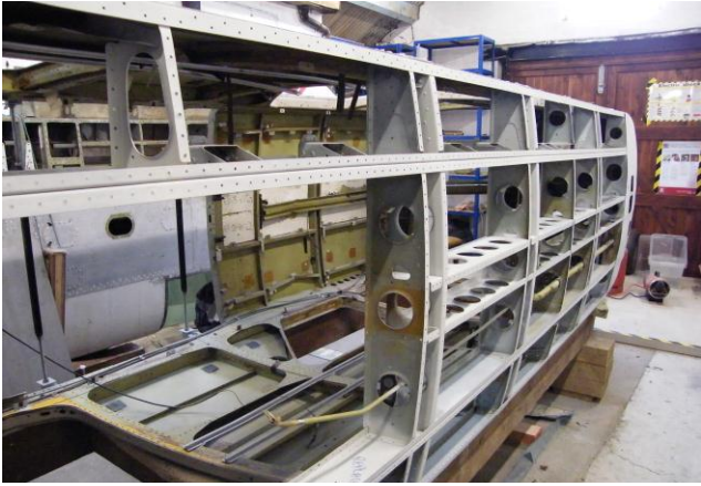
View of the refurbished under-floor frame structure
