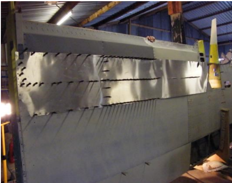
The new port outer rear bay lower wing skin is located with several skin clips and the remaining rivet fixing holes are drilled through.
