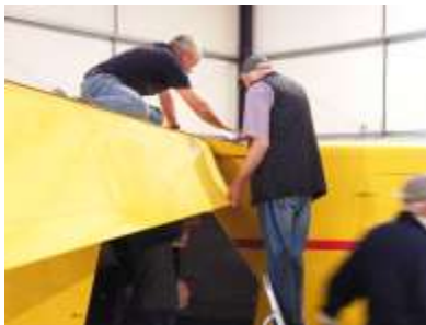
Installation of controls and flap drive motor July/August
