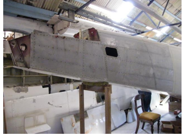
Rear starboard side view showing replacement skinning and repaired top corner section.
