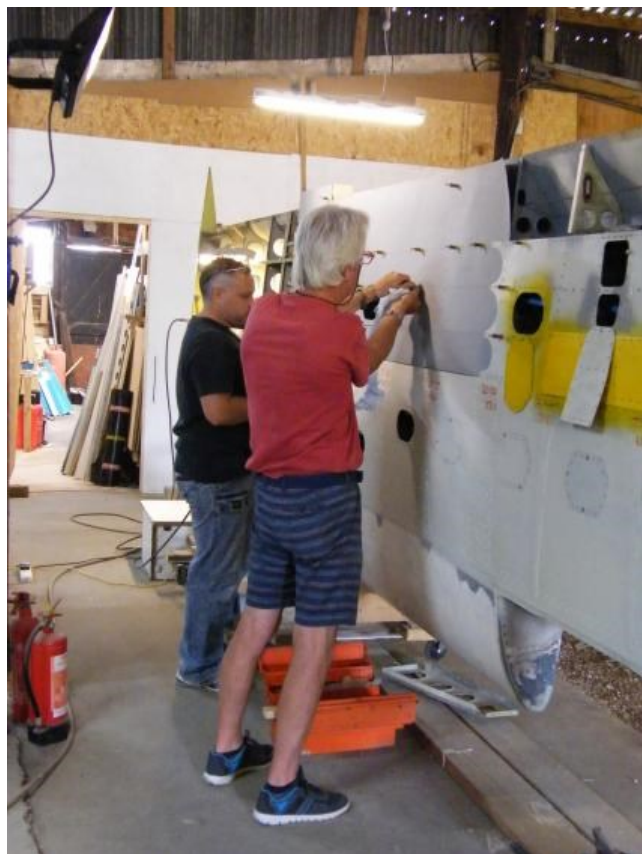
Patrick Gallagher and Steve Cooley in the process of installing the refurbished starboard wing top surface skin section with skin clips prior to it being riveted in place.
