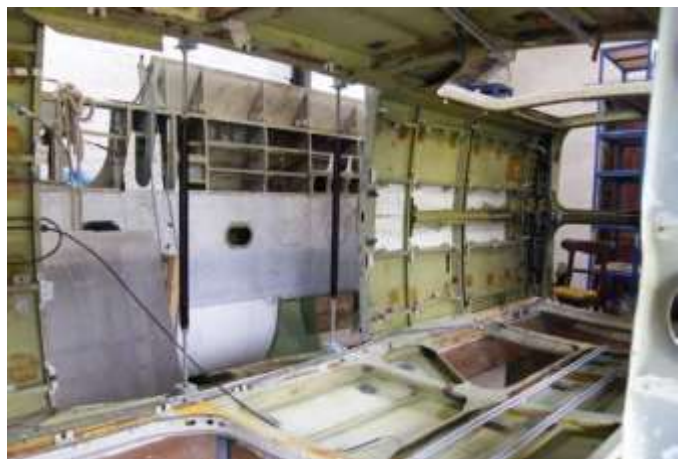
Wing pick up point tie bars were made and installed by Tim Barton at an early stage of the fuselage restoration work.
