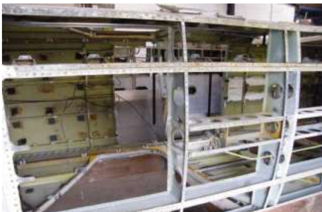
Damaged underfloor intercostals were removed for repair.
