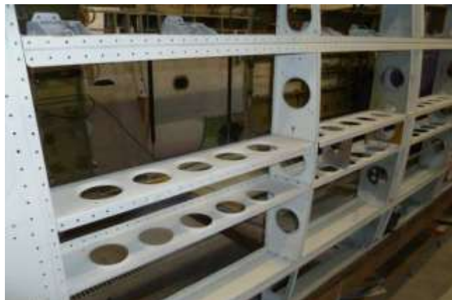
Repaired intercostals back in place and sprayed with etch-prime.
