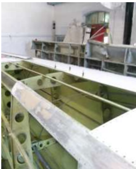
Fuselage aft roof skin slit fore and aft showing damaged starboard side removed. Also showing replacement upper corner skin in place.
