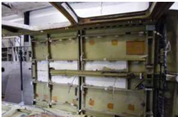
Damage to internal roof structure and top skin.
