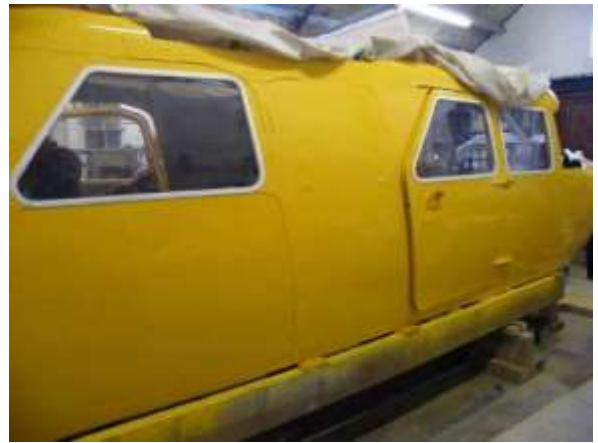
Starboard side window glazing installed.
