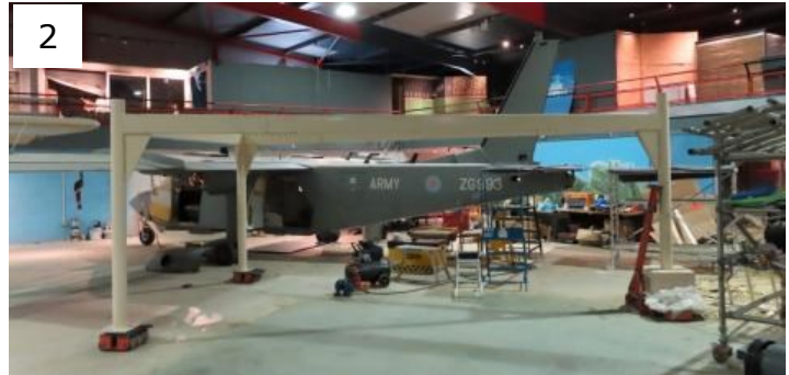
2 - Support structure on skates being moved into position.
