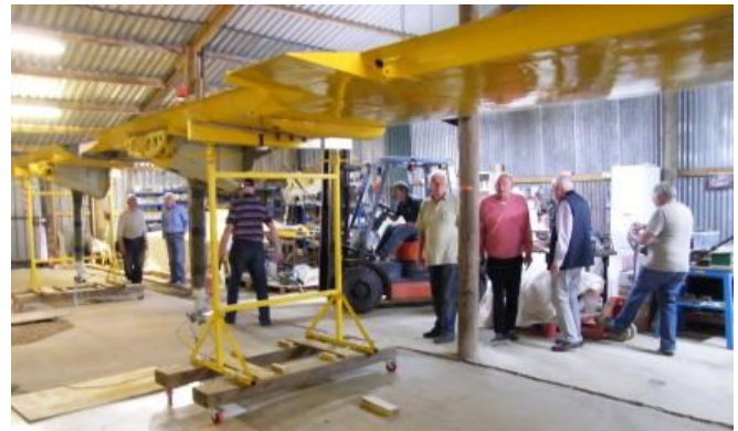
Left: First the fork lift had to be driven into the workshop and positioned for the lift.
