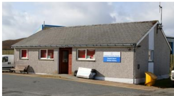
Tingwall Airport terminal building.
