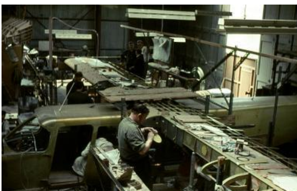
BN-2 prototype under construction in the hangar at Bembridge Airport early 1965.
