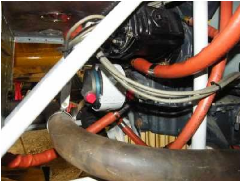
Vacuum Pump installed in place.
