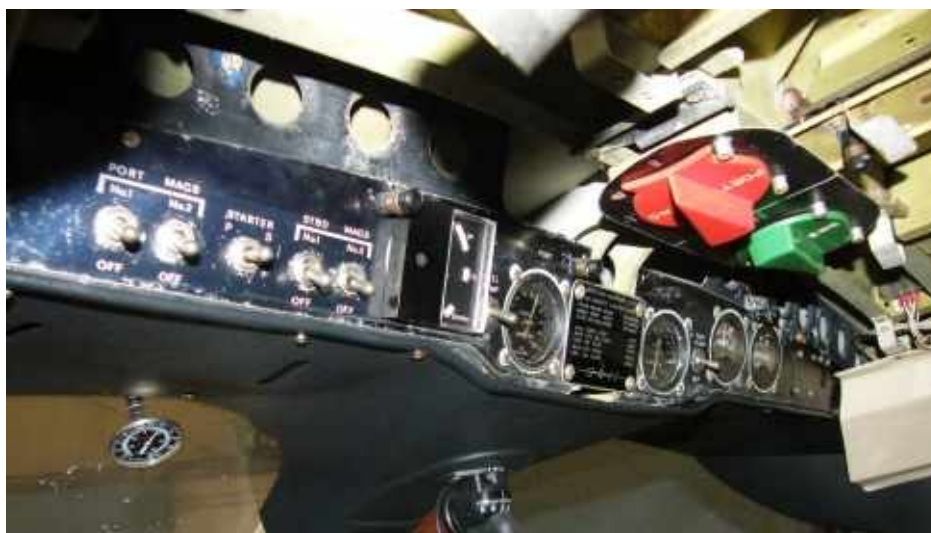
Overhead instrument panel and controls as installed
