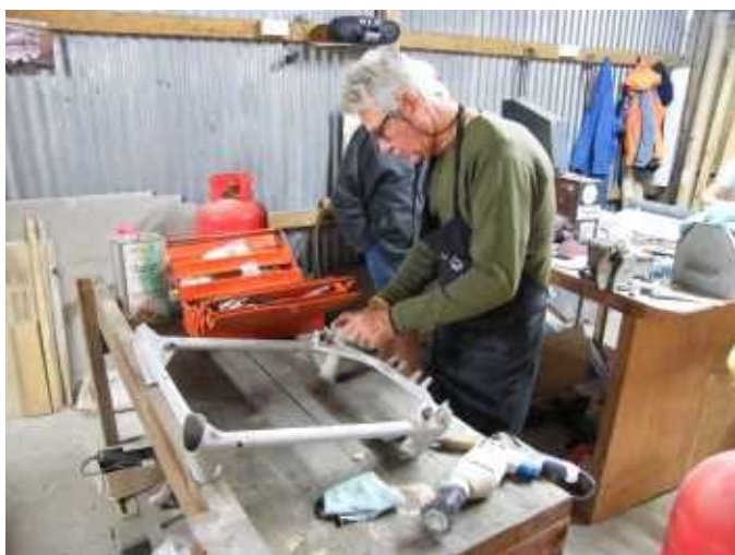
Patrick Gallagher refurbishing one of the Main Engine Frames.
