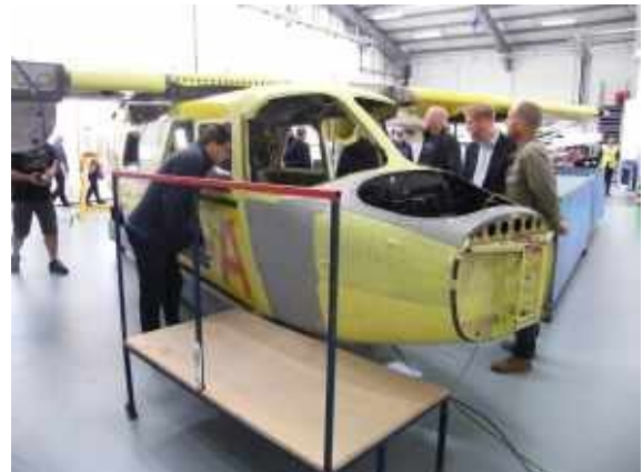
View of Islander G-BKJM showing new nose section installed during the rebuild process (BNAPS).
