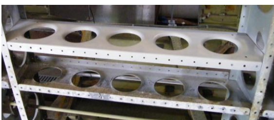
View of "cleaned up" frame section
