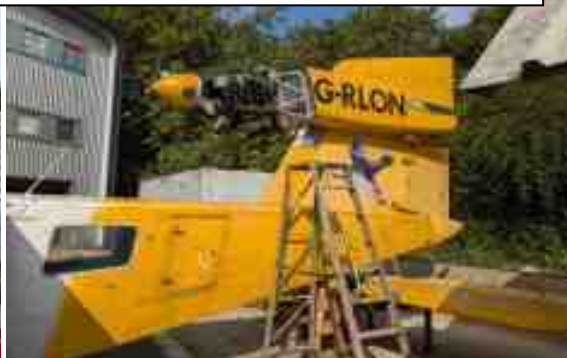
(right) Tail engine in process of being secured during installation
